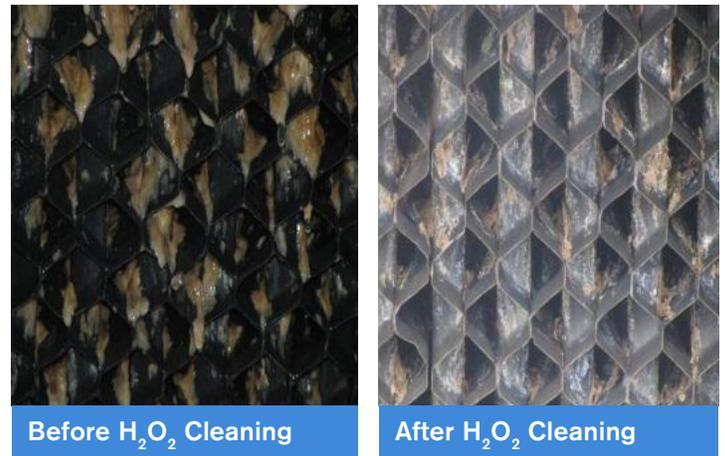
Five hours after hydrogen peroxide was added to the tower, the turbidity stabilized and the peroxide level in the bulk water was down to <20 ppm, at which point the water was evacuated from the tower to remove the solids from the system.
