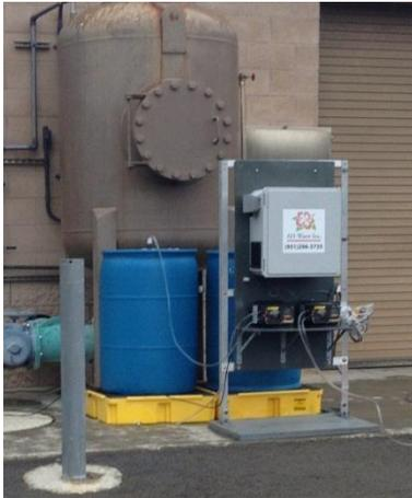
The second subsystem is the chemical injection/mixing/controls (IMC) module which is placed in the wetwell to ensure accurate dosing and complete mixing (Figure 5). The module includes a submersible pump that draws in wastewater, mixes in the acid, and distributes the pH-adjusted water throughout the wetwell. Acid feed is controlled by two separate pH probes situated in different parts of the wetwell, and nitrite feed is paced to the influent wastewater flow.
