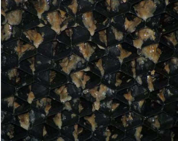
**Figure 25. Close-up of underside of fill pack prior to peroxide cleaning showing goeey slime buildup.**
