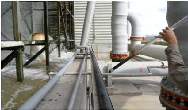
**Figure 32. Tower basin during cleaning with "sludge judge".**
