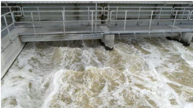
**Figure 31. Counterflow combined cycle power plant tower screen pit during cleaning.**
