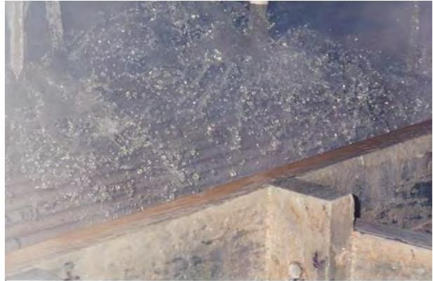
**Figure 13. Tube bundle totally white with calcium carbonate under a spray nozzle near the start of the cleaning procedure**
