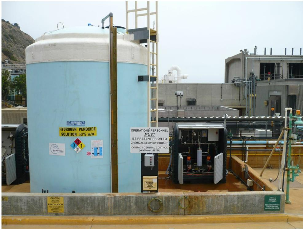
**Figure 6: Headworks Hydrogen Peroxide Feed System**
